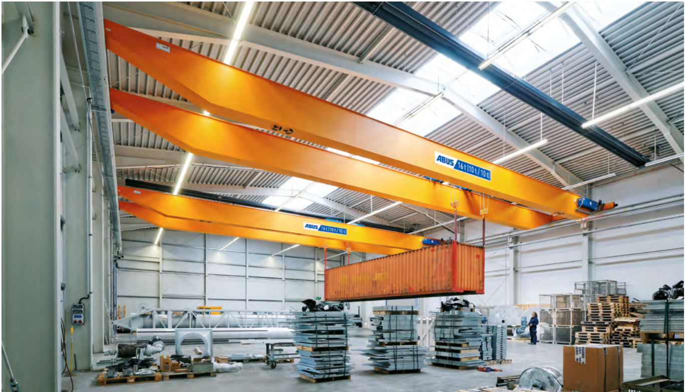
When transporting long and bulky goods, two cranes working simultaneously in tandem ensure risk-free load handling
