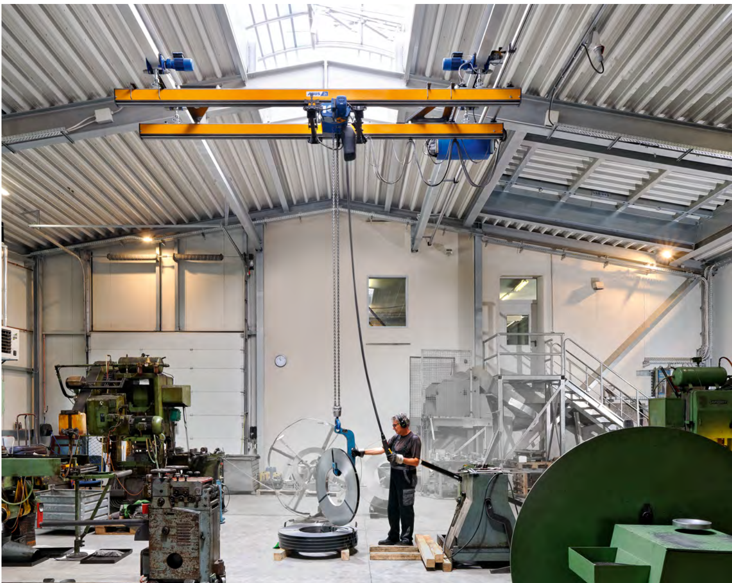
Mobile due to powered trollies on steel support beams
